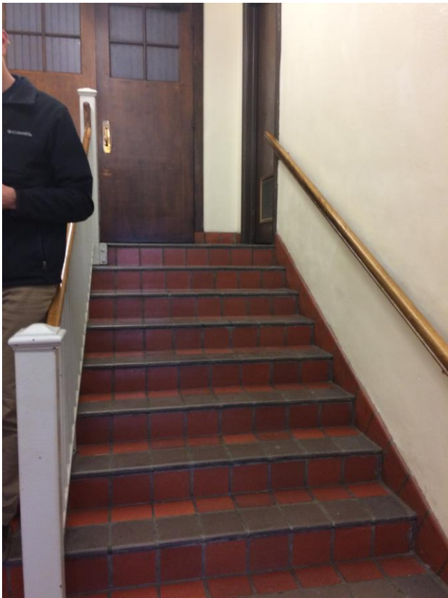
Stairs at gym entrance prohibit ADA access
