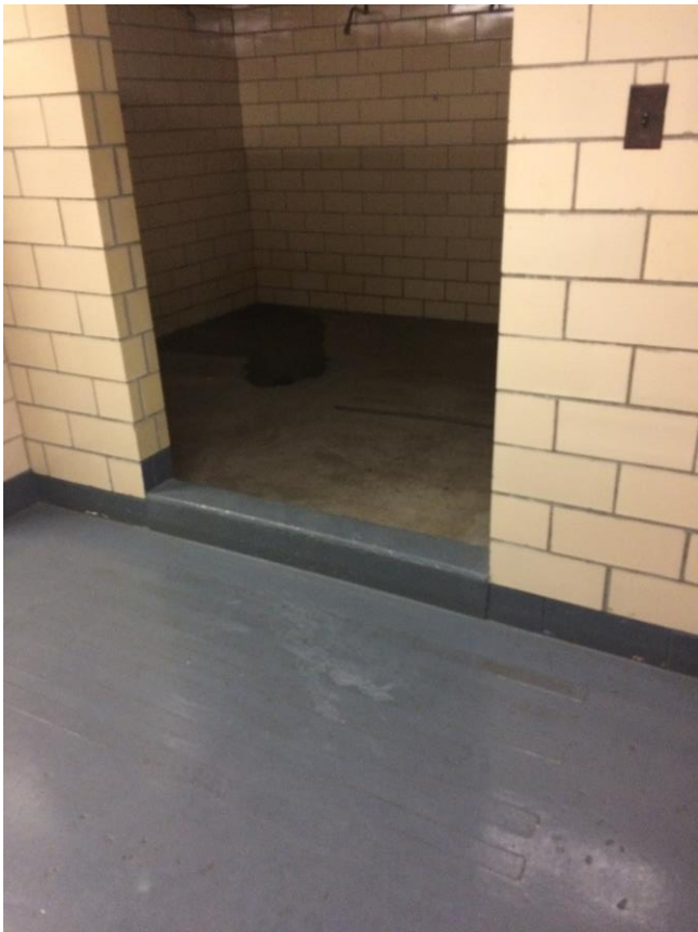
ADA barrier in shower room
