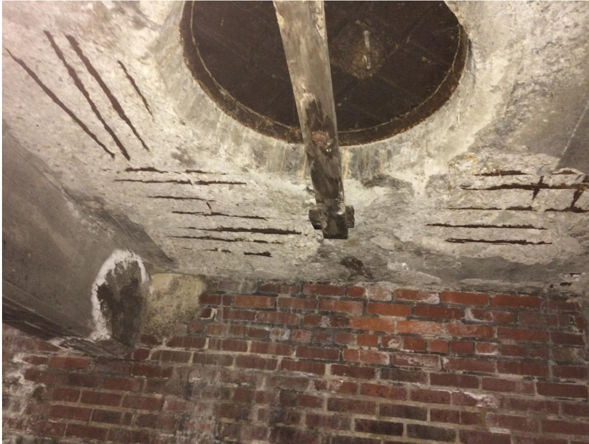
Concrete roof deck erosion – exposing steel
