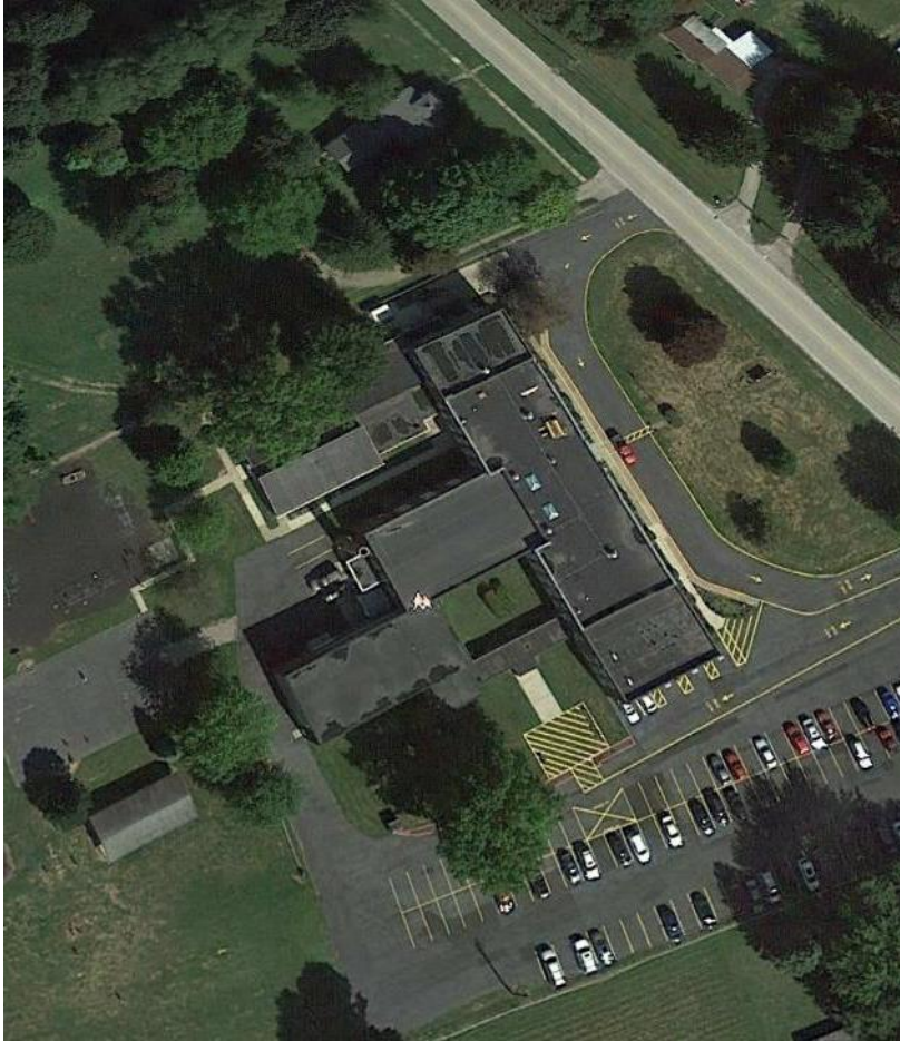
Roofs need replacement – additional insulation needed to meet LEED
