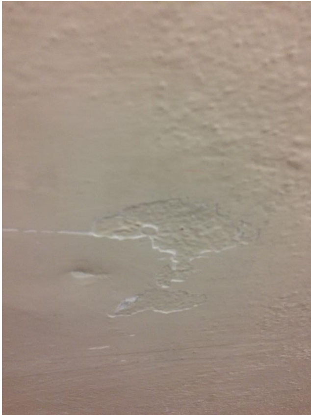
Plaster repairs/refinishing needed
