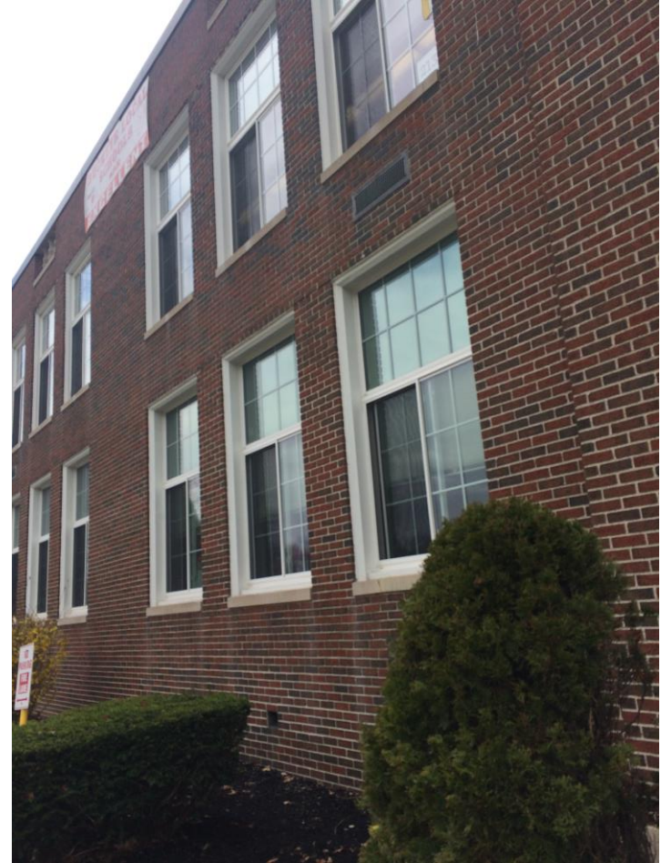
Windows are in poor condition
