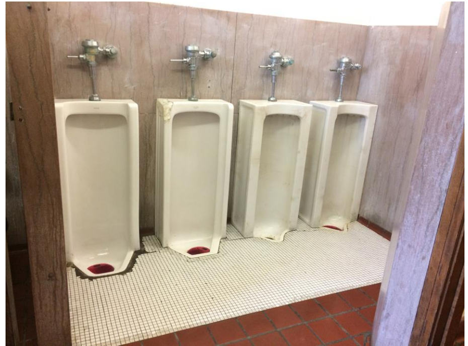
Removal of floor mounted urinals will require patching
